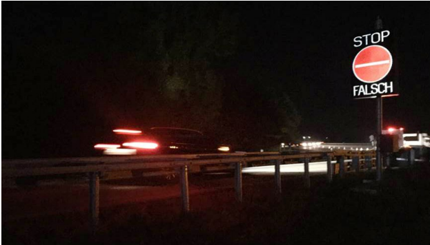
≡ A 9 wrong-way driver warning system
