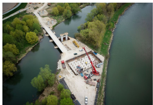
↗ St 2124, Plattling roundabout, new construction of the Isar bridge with lifting of the first steel parts at the abutment
