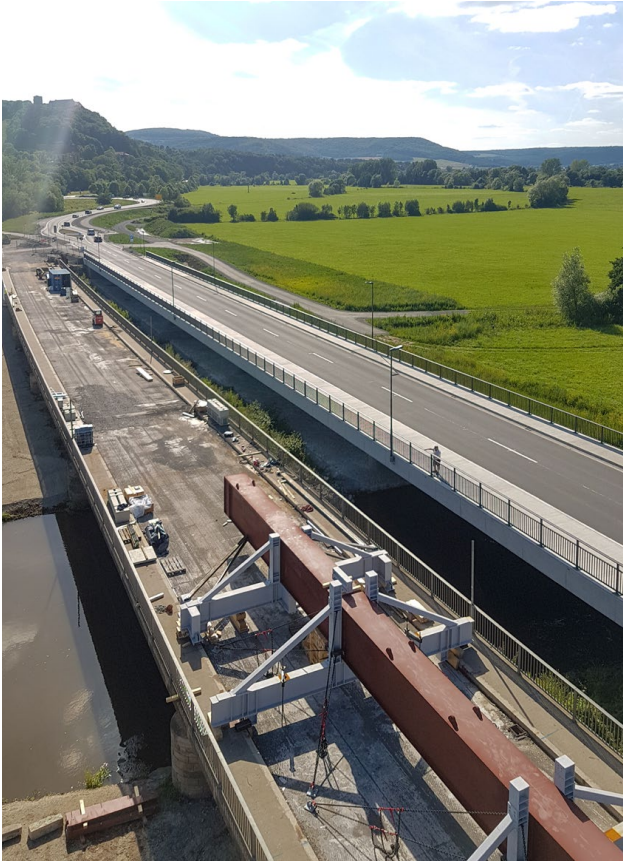
Old and new Saalebrücke Hammelburg with test stand on the old bridge
