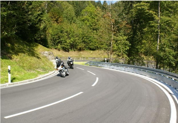
➤ Bend with retrofitted underrun protection
