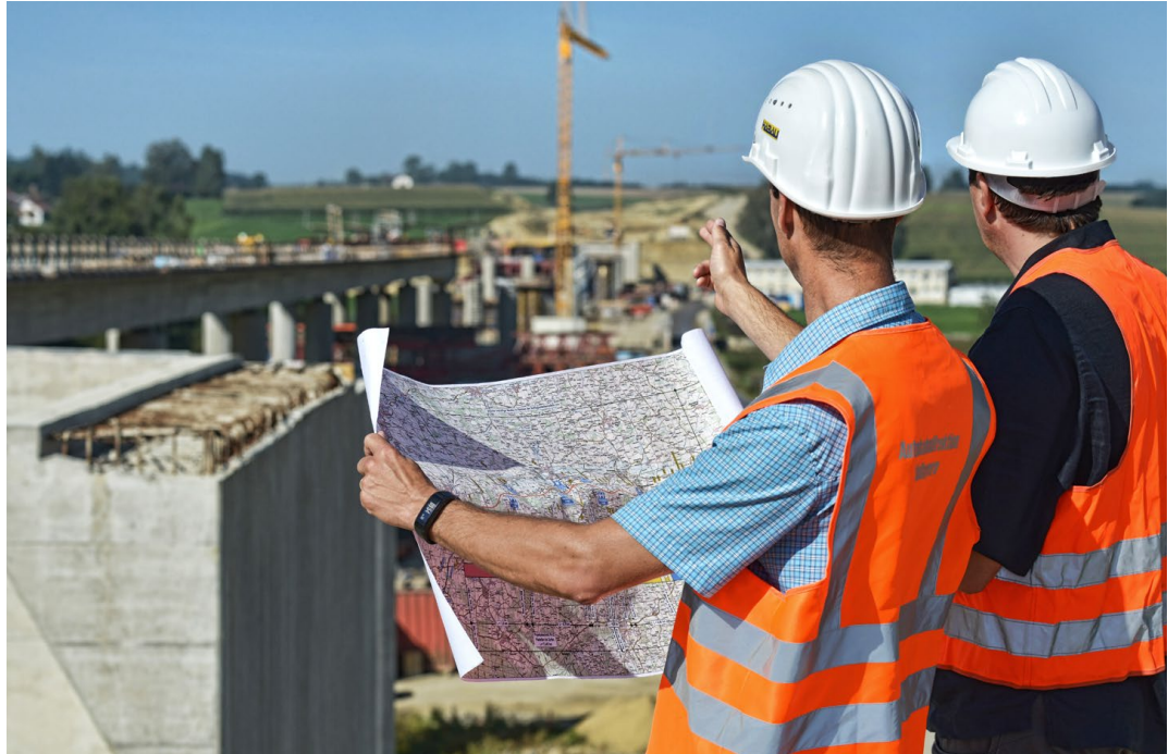
» A 94, construction management on a motorway construction site
