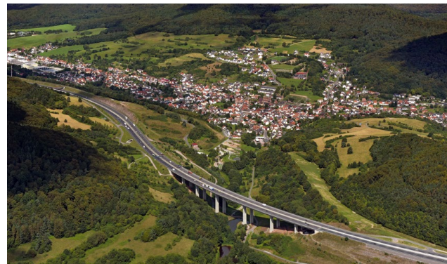
➤ A 3, Kauppen bridge at Waldaschaff; the new route has been moved up to 300 metres
