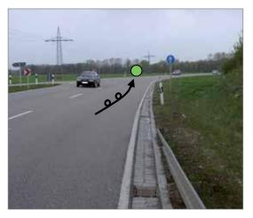
Both the radius and the transverse slope decreased suddenly in the bend, which resulted in an accumulation of single-vehicle accidents.
