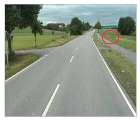
The installed signpost improves the visibility of the intersection on the major road. **BUT:** The font size of the signpost is not sufficient. A left-turning lane is still lacking.
