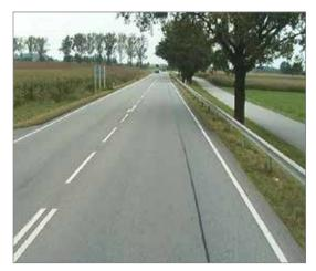
Passive safety was increased by installing a steel crash barrier. This also increased the protection of cyclists on the bicycle path running parallel to the road.
