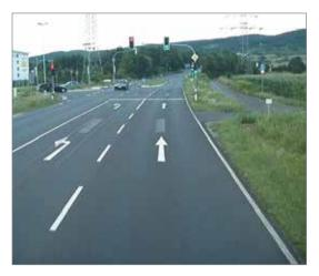
A traffic light system provides sufficiently long time gaps in the main flow for safe turning into/ crossing of the major road from the low-traffic minor road. At the same time, the traffic-actuated light signal control system provides for high throughput.
