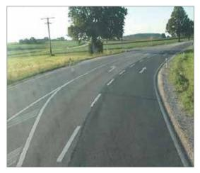
The added left-turn lane improves the visibility of the intersection on the major road and enables left turns without any danger to following straight-through traffic.
