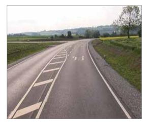
The added left-turn lane improves the visibility of the intersection. **BUT:** A channelizing island (droplet shape) on the minor road and signposting is still lacking.
