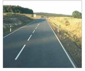
The changed layout of the road has no turning line and makes the further course of the road towards the right clear.
