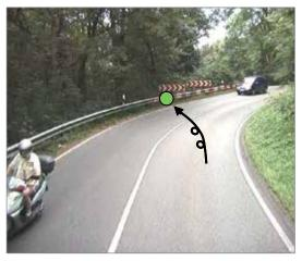
The traffic guidance equipment was insufficient to indicate the direction of the bend, which promoted single-vehicle accidents.
