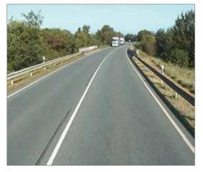
The solid line centre road marking prohibits overtaking and thus reduces the speed level.
