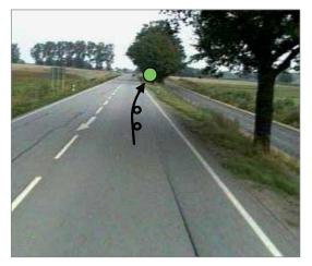
The road was in a poor condition. In addition, there were trees at the edge of the road. Departure accidents where vehicles collided with the trees at the edge of the road had very severe consequences.
