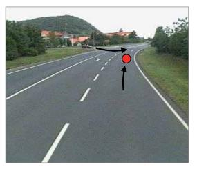
The intersection was hard to see from the minor road, which caused severe accidents when vehicles turned into the major road.
