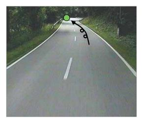
The direction of the bend was hard to see. High speeds led to single-vehicle accidents.
