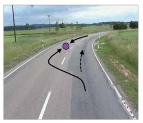
The course of the road was hard to see which is why the curvature of the road was underestimated. This repeatedly caused accidents involving longitudinal traffic (rear-end and head-on collisions) when overtaking. Measure
