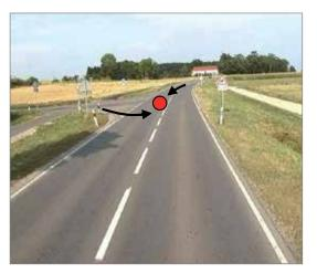
The intersection was hard to see in the dark. In addition, drivers drove too fast, which made it difficult for vehicles coming from the minor road to turn into the major road (short time gaps in the main flow). Measure
