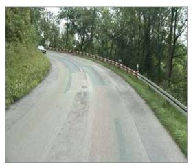
Traffic guidance equipment installed on top of the steel crash barrier makes it easier to see the direction of the bend.
