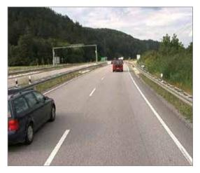
The extension of the road to a dual carriageway separates the carriageways for opposite travelling directions and provides for safe overtaking and increases capacity.
