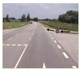
The large waiting area on the minor road incited drivers to enter the major road too quickly, which caused conflicts when decelerating and resulted in rear-end collisions. Measure
