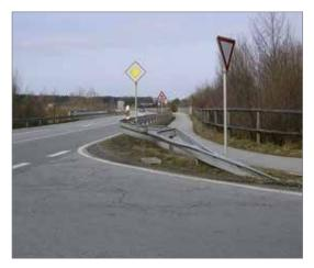
Visibility for traffic turning into the major road was improved by removing the vertical extension rail.
