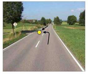
The intersection was hard to see and, together with the straight road layout, this promoted high driving speeds resulting in severe accidents with turning-off vehicles.
