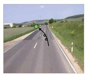
The condition of the road suddenly deteriorated at the end of the extension work, which promoted single-vehicle accidents.
