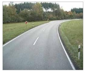
Individually placed bend chevrons indicate the direction of the bend. **BUT:** The road is still in poor condition.
