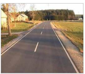
A bend was removed in the new road layout to make the further course of the road towards the right clear. In addition, the cross-section was widened, the road was resurfaced and its marking was renewed.
