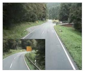
The destination sign with arrows indicating the directions is located before the bend and signals the intersection well in advance. This also improved the visibility of drivers turning into the major road.
