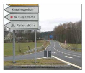
Visibility for traffic turning into the major road was improved by moving the signposts up, lowering the marker board and removing the marker post.
