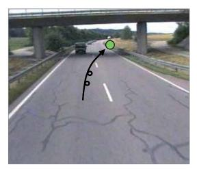
The straight layout of the road incited drivers to drive very fast. However, visibility was insufficient for overtaking due to the bridge. Aborted overtaking manoeuvres caused drivers to lose control of their vehicle.
