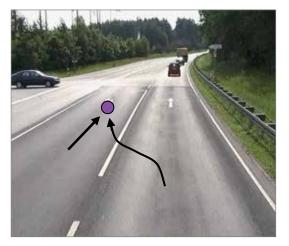
High driving speeds and high traffic volumes on the major road incited drivers to initiate risky lane changes ahead of the intersection which caused rear-end collisions with following vehicles. Measure
