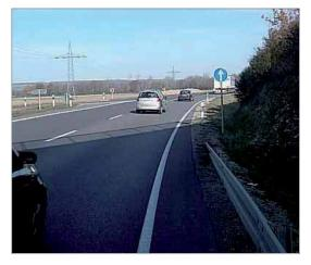
The new layout of the right road edge with a continuous radius and an increased consistent transverse slope eliminated the accident blackspot.
