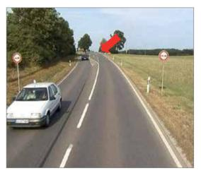
High speeds on the major road made it difficult to turn into the major road from the minor road (short time gaps) causing the vehicles turning into the road to collide with vehicles having the right of way.
