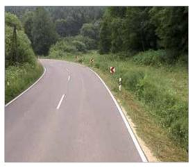
Additional individually placed bend chevrons make the direction of the bend clearer. **BUT:** Visibility is still limited by the vegetation in the inner bend.
