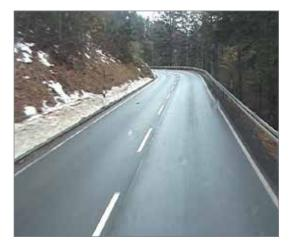
Thanks to the renewed wearing course, the road is again in a good condition. **BUT:** Visibility is still very limited due to the slope in the inner bend.
