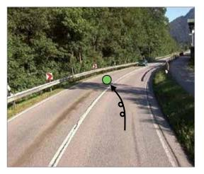
The transverse slope and the condition of the road were inadequate. In addition, the layout of the road was discontinuous, repeatedly resulting in single-vehicle accidents when the road was wet.
