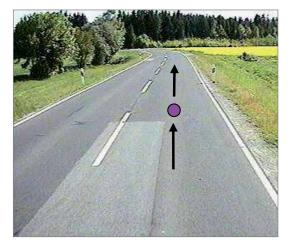
The layout of the road was discontinuous and the road was in a poor condition, which promoted rear-end collisions when the road was wet.
