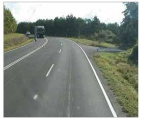
The double solid line centre road marking makes the lane limits, the course of the road and the three-lane, single-carriageway layout of the road clearer.
