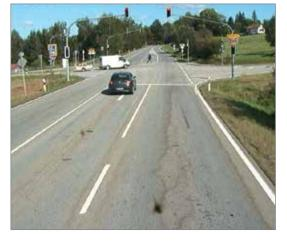
A separate left-turn phase "protects" road users turning left into the minor road from encountering oncoming traffic.
