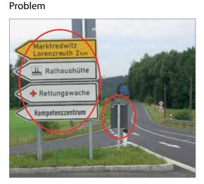
The visibility splay (range of vision required for a driver to safely turn into a major road from a stop) at the intersection was insufficient. Accidents with vehicles having the right of way occurred as vehicles turned into the major road despite of bad visibility.
