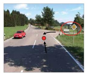
The visibility splay (range of vision required for a driver to safely turn into a major road from a stop) at the intersection was insufficient for both passenger vehicles and lorries. Accidents with vehicles having the right of way occurred as vehicles turned into the major road despite of bad visibility.
