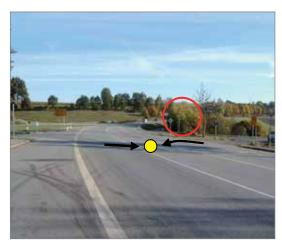
The vegetation on the side of the road's bend limited the visibility of vehicles coming from the direction of the minor road so that drivers concentrated on gaps between the vehicles in the flow on the major road and collided with oncoming vehicles when turning left.
