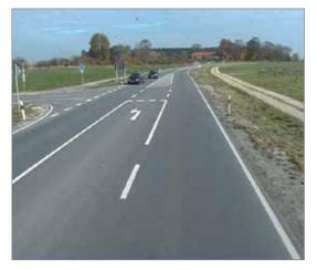
The added left-turn lane improves the visibility of the intersection, especially in the dark. **BUT:** A channelizing island (droplet shape) on the minor road is still lacking.
