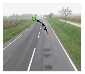
The road was in a poor condition and the layout of the road was discontinuous. As the road sloped up, the course of the road behind the slope was hard to see, which promoted single-vehicle accidents.
