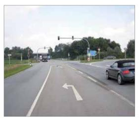
A traffic light system provides sufficiently long time gaps in the main flow for safe turning into/ crossing of the major road. In addition, the separate left-turn phase provides increased safety when turning.
