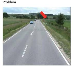
The intersection was hard to see. Drivers overtook other vehicles before the intersection, which caused them to recognize vehicles turning too late and the following traffic collided with the vehicle's rear end. Measure
