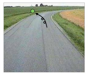
Due to the lack of marking it was hard to see the direction of the bend, especially at night, which promoted single-vehicle accidents.
