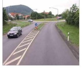
The conversion into a roundabout reduces the speed level at the intersection and makes turning into/crossing the major road easier. The lighting of the roundabout, especially outside of lit built-up areas ensures better visibility at night.
