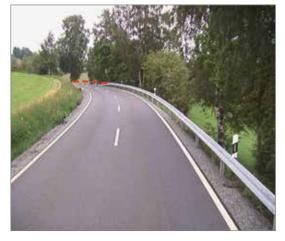
Passive safety was increased by means of a steel crash barrier.
