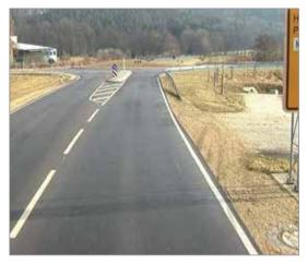
The conversion into a roundabout reduces the speed level at the intersection and makes turning into/crossing the major road easier (reduction of conflict points).
