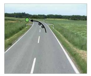
The layout of the road was discontinuous and the double bend could not be seen, which promoted single-vehicle accidents.
