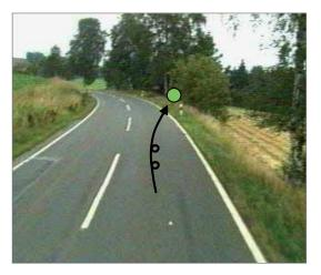
The direction of the bend was hard to see. In addition, there were trees at the edge of the road. Single-vehicle accidents where vehicles collided with the trees in the outer bend had severe consequences.
