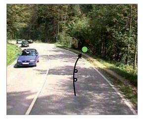
The road layout was discontinuous. In addition, there were trees at the edge of the road. The direction of the bend was hard to see, which promoted single-vehicle accidents that had severe consequences where vehicles collided with the trees.
