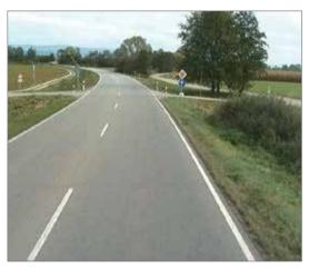
Visibility for traffic turning into the major road was improved by cutting back the vegetation. BUT: The vegetation has to be cut back at regular intervals.
