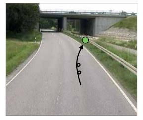
The centre road marking was in a poor condition and could hardly be seen at all. In addition, it was hard to see the further direction of the road due to a bridge, which promoted singlevehicle accidents.
