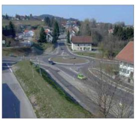
A roundabout unambiguously determines the right of way situation and reduces the speed level and thus the severity of accidents. BUT: Destination signs on the centre island are still lacking.
