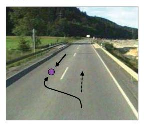
The road section provided few opportunities for overtaking while the volume of traffic was quite high. Overtaking despite short time gaps in incoming traffic repeatedly caused severe accidents involving longitudinal traffic (rear-end and head-on collisions).
