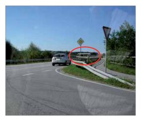
The visibility splay (range of vision required for a driver to safely turn into a major road from a stop) at the intersection was insufficient for passenger vehicles. Accidents with vehicles having the right of way occurred as vehicles turned into the major road despite of bad visibility.
