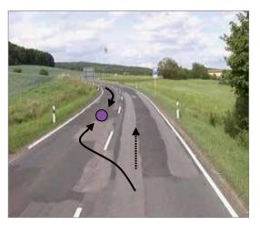
The direction of the bend (turning line) was hard to see. Overtaking manoeuvres in the area of the bend resulted in head-on collisions with severe consequences.
