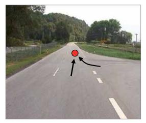
The stop line was no longer visible causing vehicles to turn into the priority road without stopping and colliding with vehicles having the right of way.
