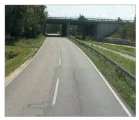
The renewed centre road marking makes the course of the road clearer. BUT: This measure could not improve the limited field of vision caused by the bridge.
