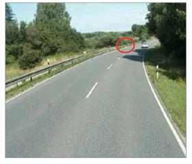
Thanks to the new wearing course, the road has more grip. In addition, the type II marking provides increased night-time visibility. **BUT:** The steel crash barrier has a gap.
