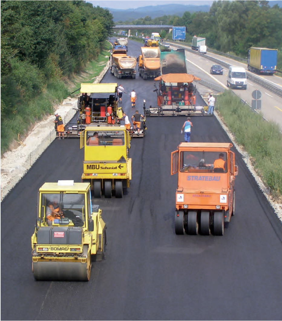
Figure 3: Pavement construction on a motorway
