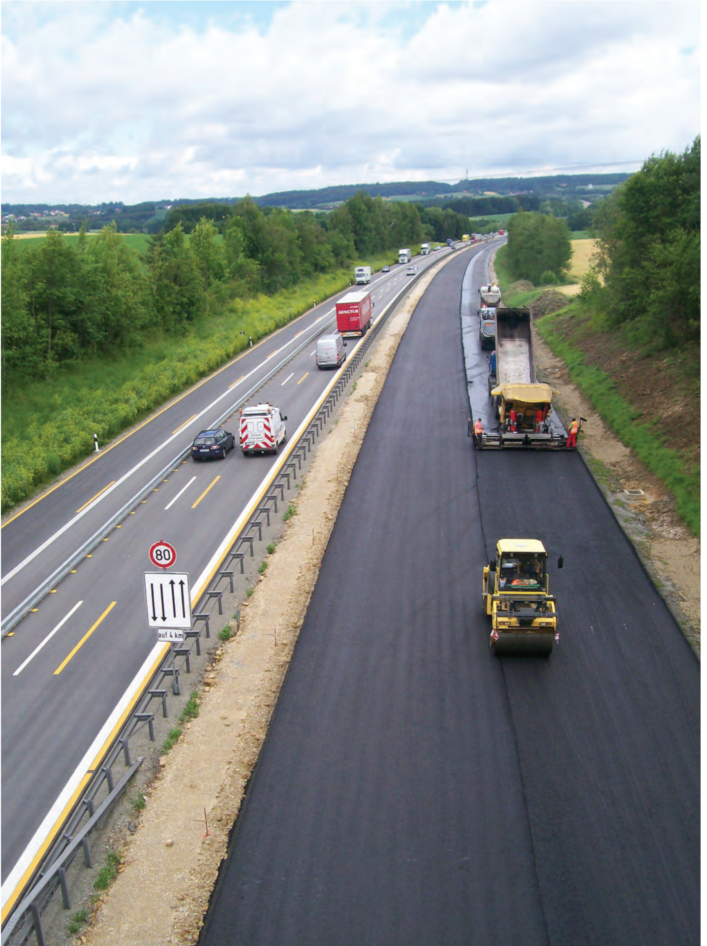
Asphalt work on a motorway
