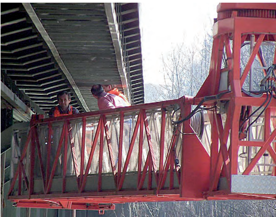
Fig. 3: Bridge inspection with underfloor device
