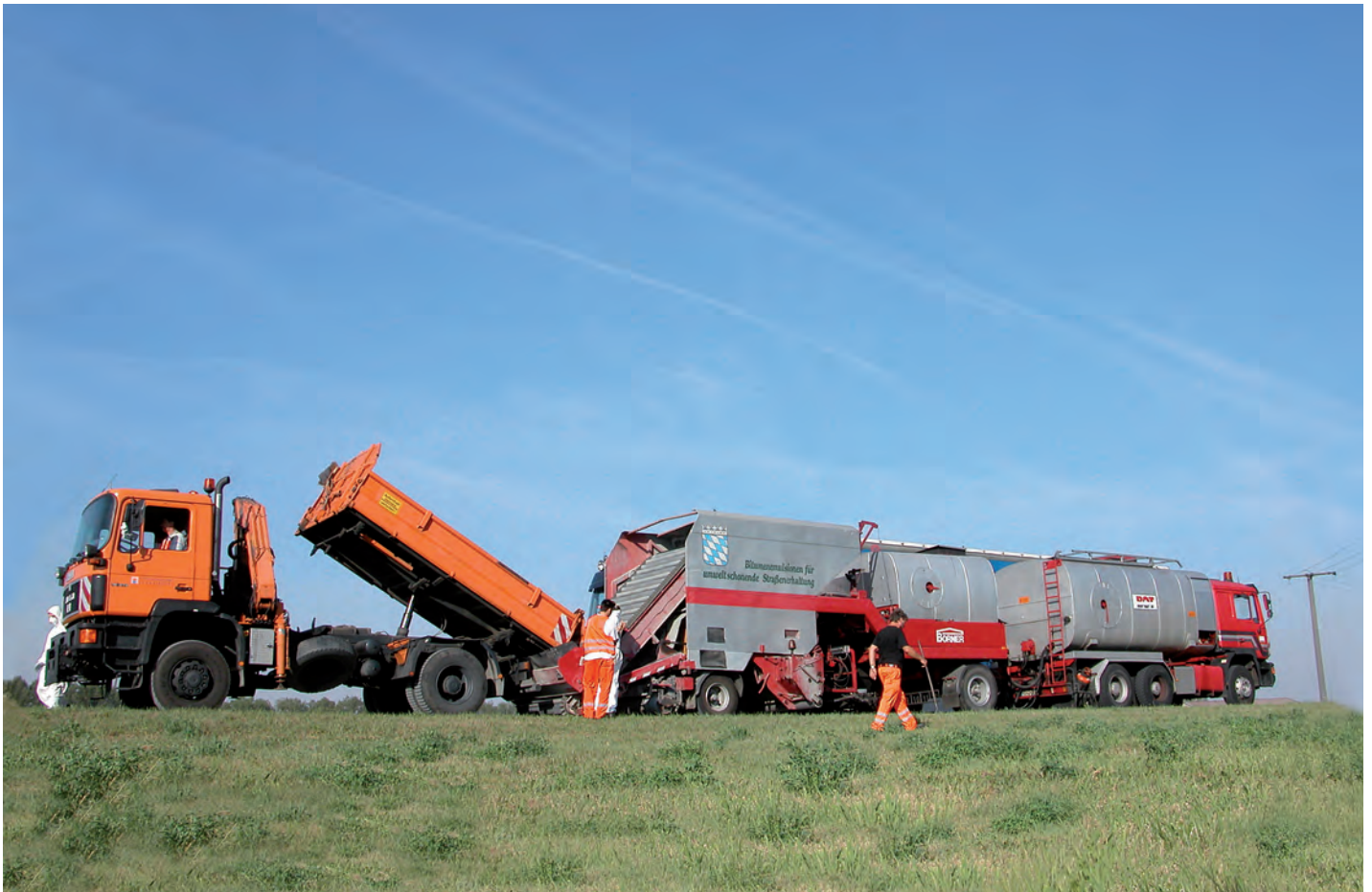
Figure 6: Maintenance measure (surface treatment)
