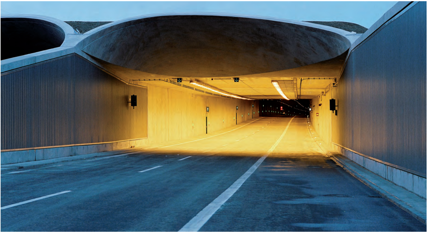
Fig. 7: A99 federal motorway, Aubing tunnel portal
